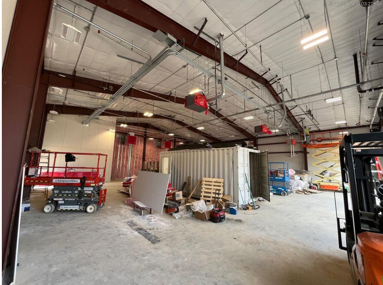
4/18/24 Apparatus bay progress overview
