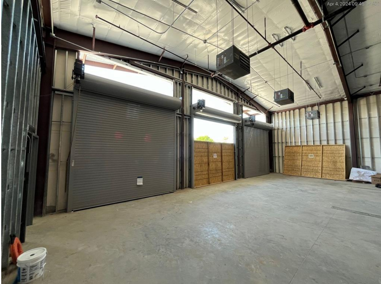
4/4/24 Apparatus bay overhead doors installed
