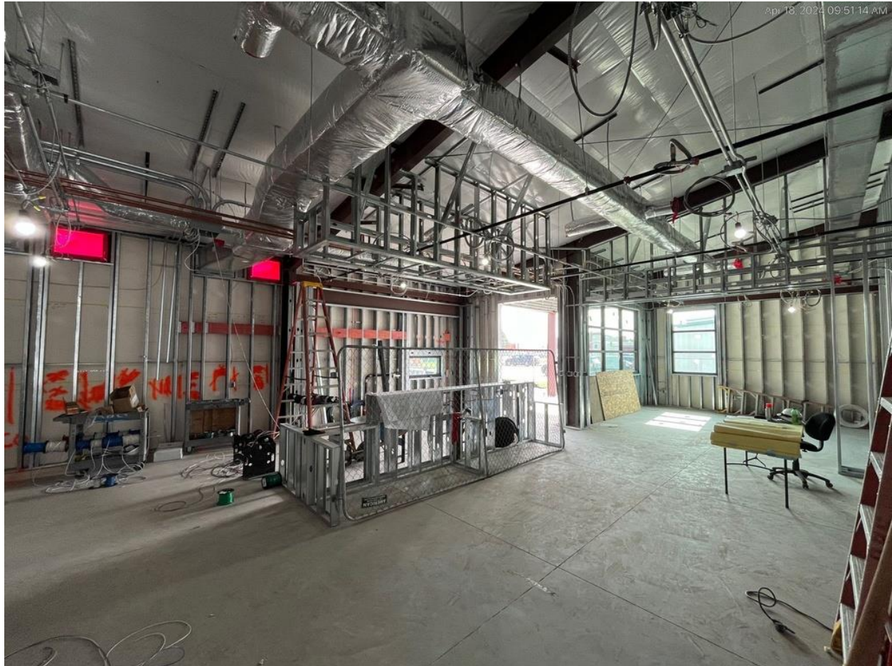
4/18/24 Kitchen progress overview
