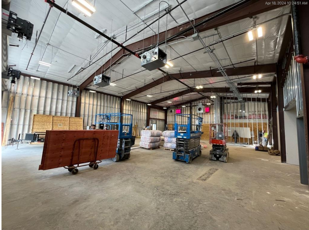
4/18/24 Apparatus bay progress overview
