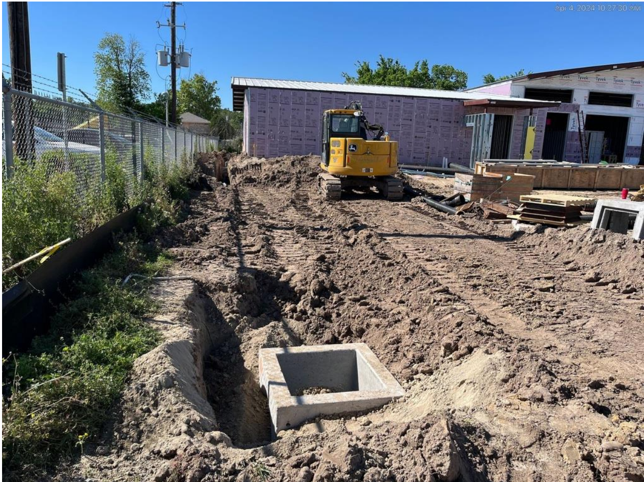
4/4/24 Site utility installation underway
