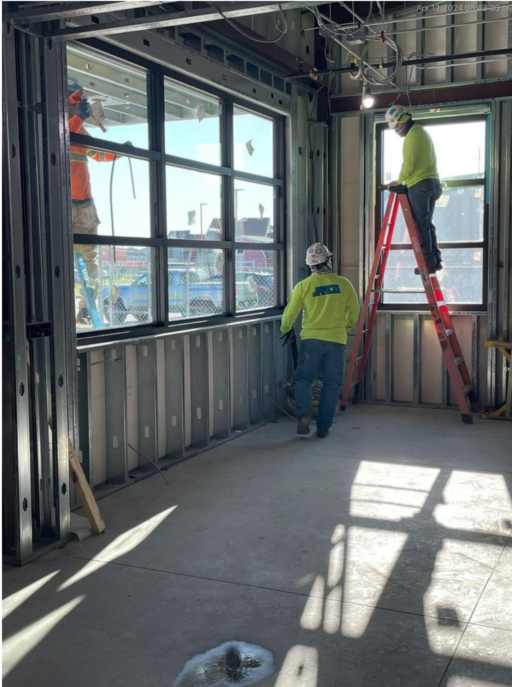
4/12/24 Window install underway
