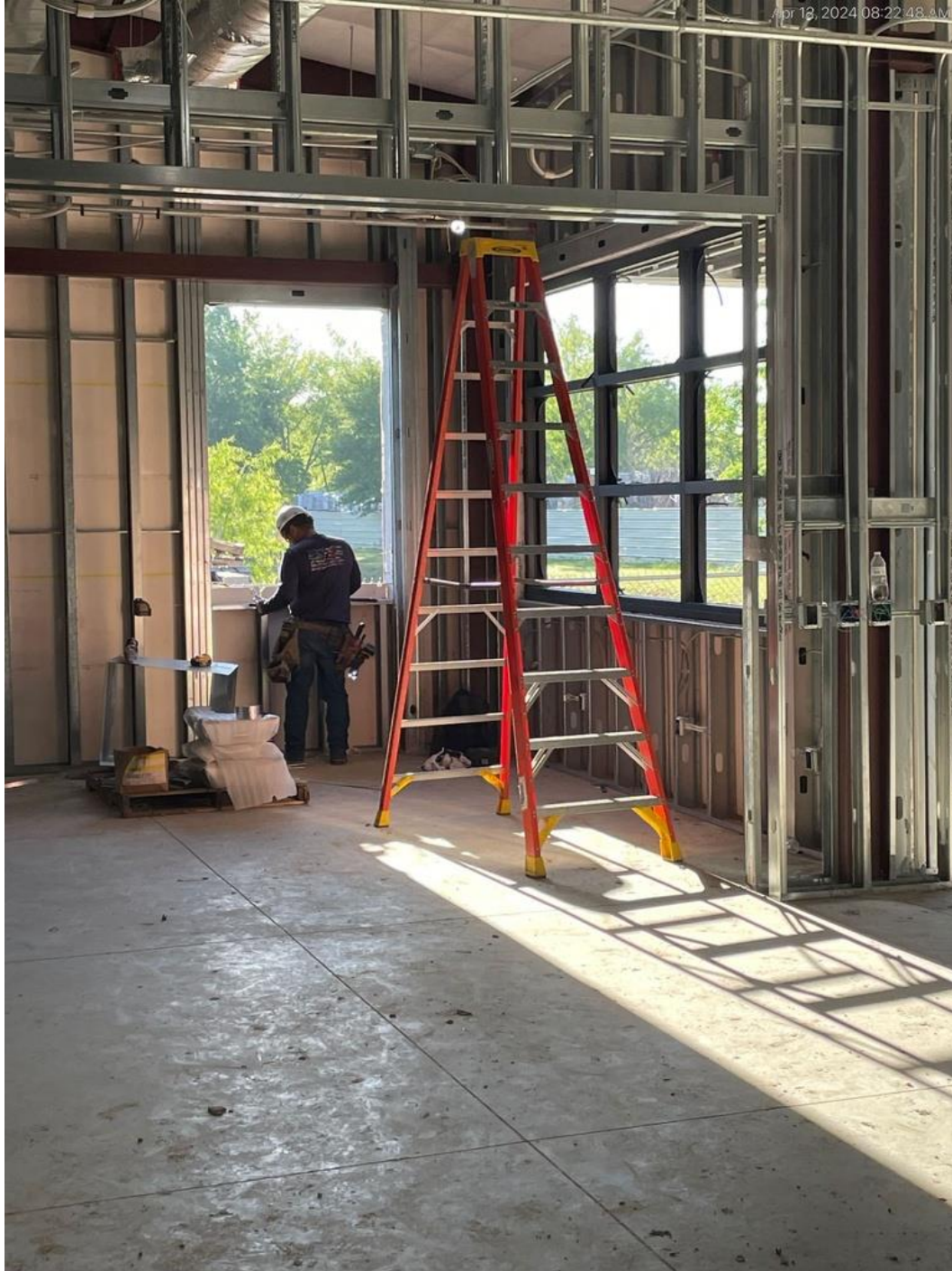
4/12/24 Window installation underway
