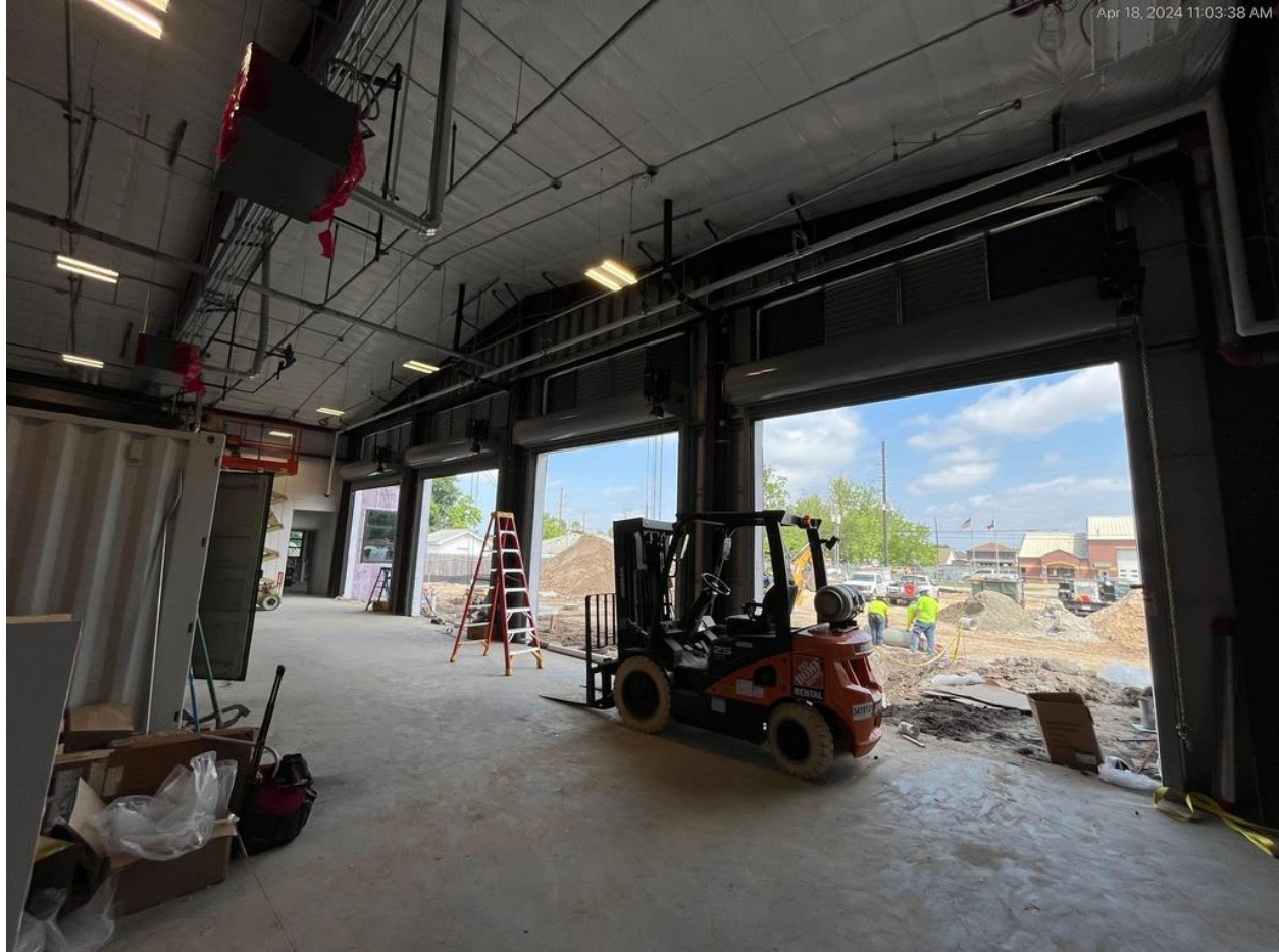
4/18/24 Apparatus bay overhead doors installed
