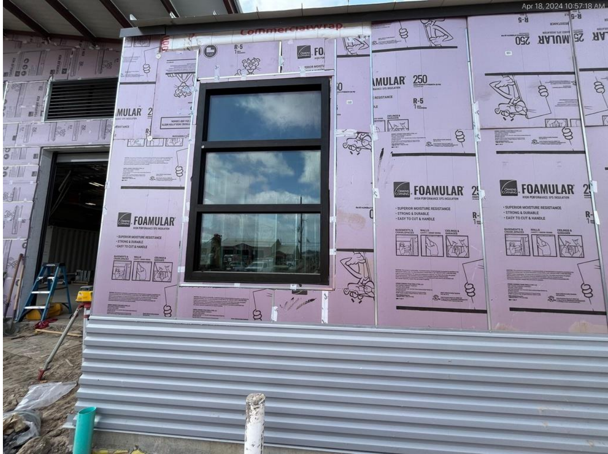
4/18/24 Mockup wall progress overview
