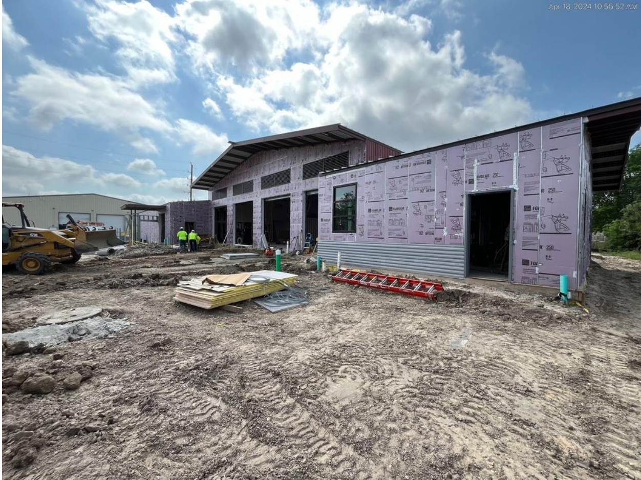
4/18/24 Building progress overview
