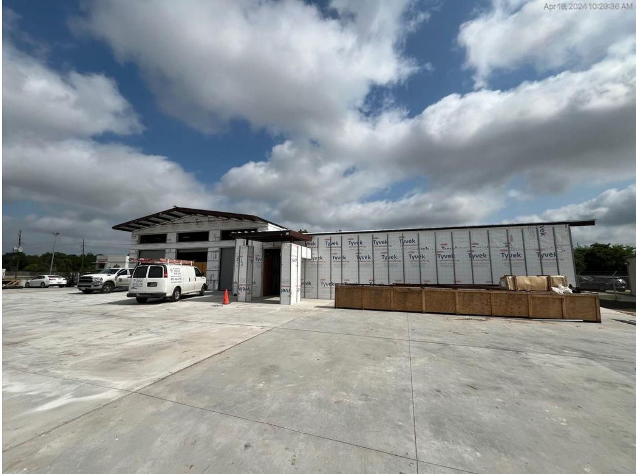
4/18/24 Building exterior progress overview
