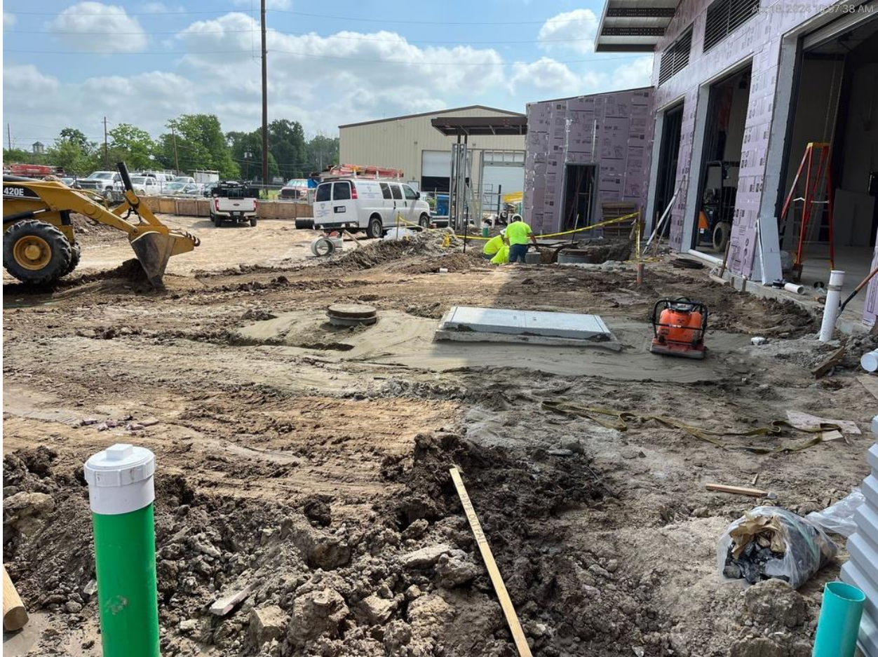
4/18/24 Grease trap and sand/oil separator being installed
