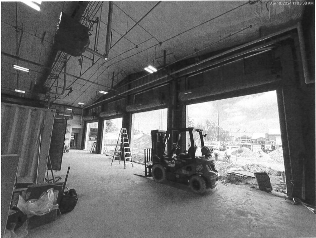
4/18/24 Apparatus bay overhead doors installed
