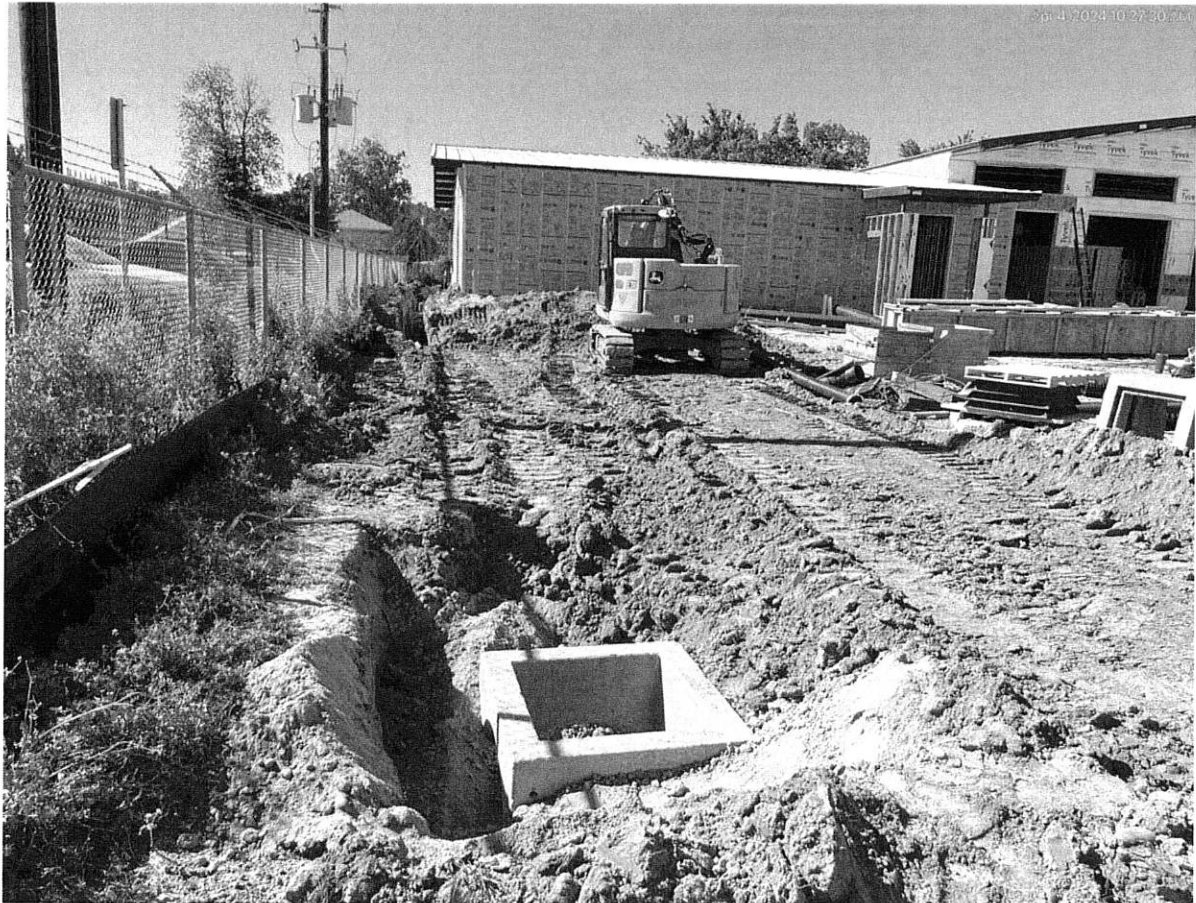
4/4/24 Site utility installation underway
