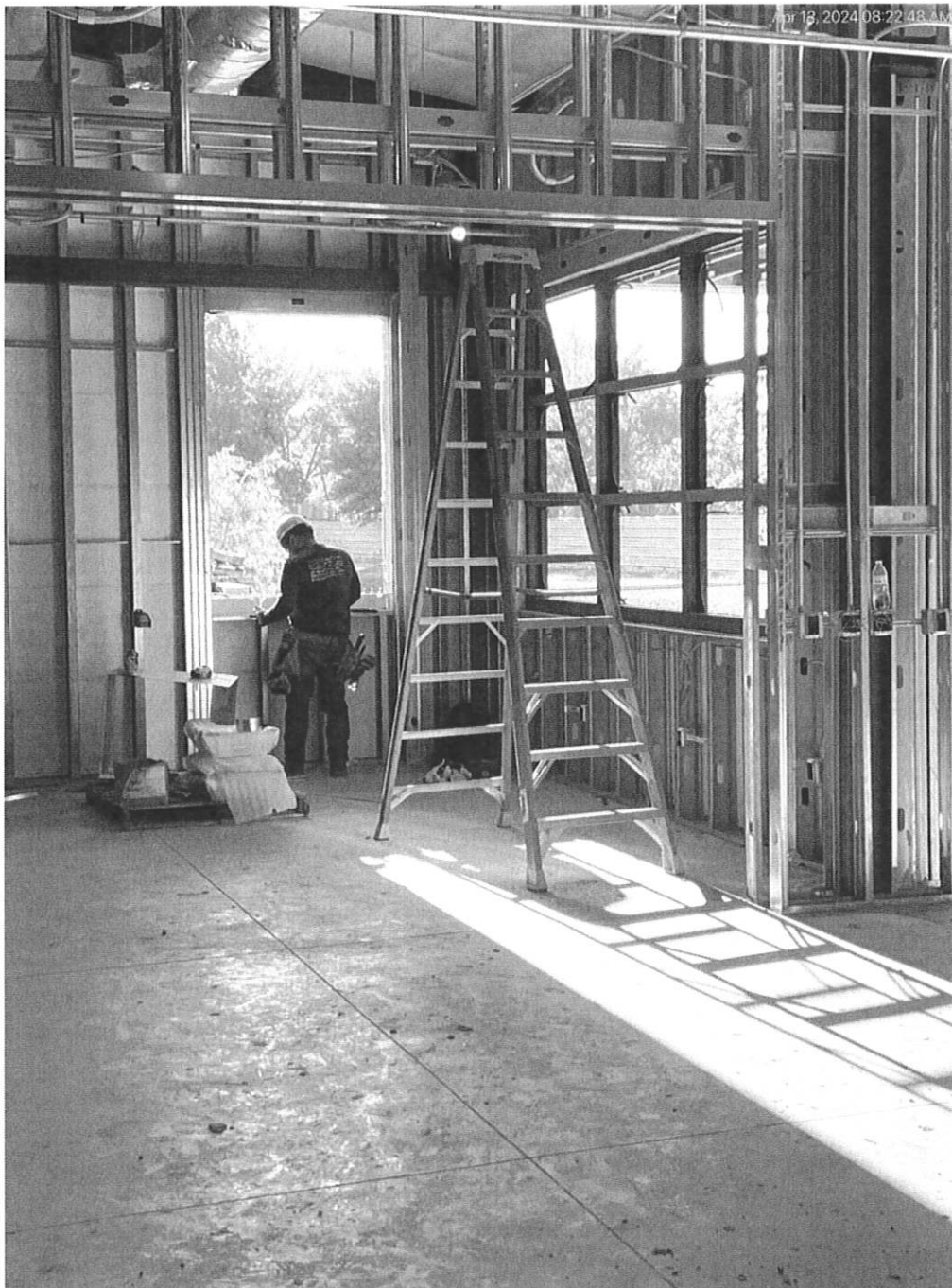
4/12/24 Window installation underway
