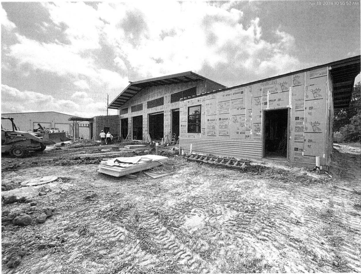
4/18/24 Building progress overview
