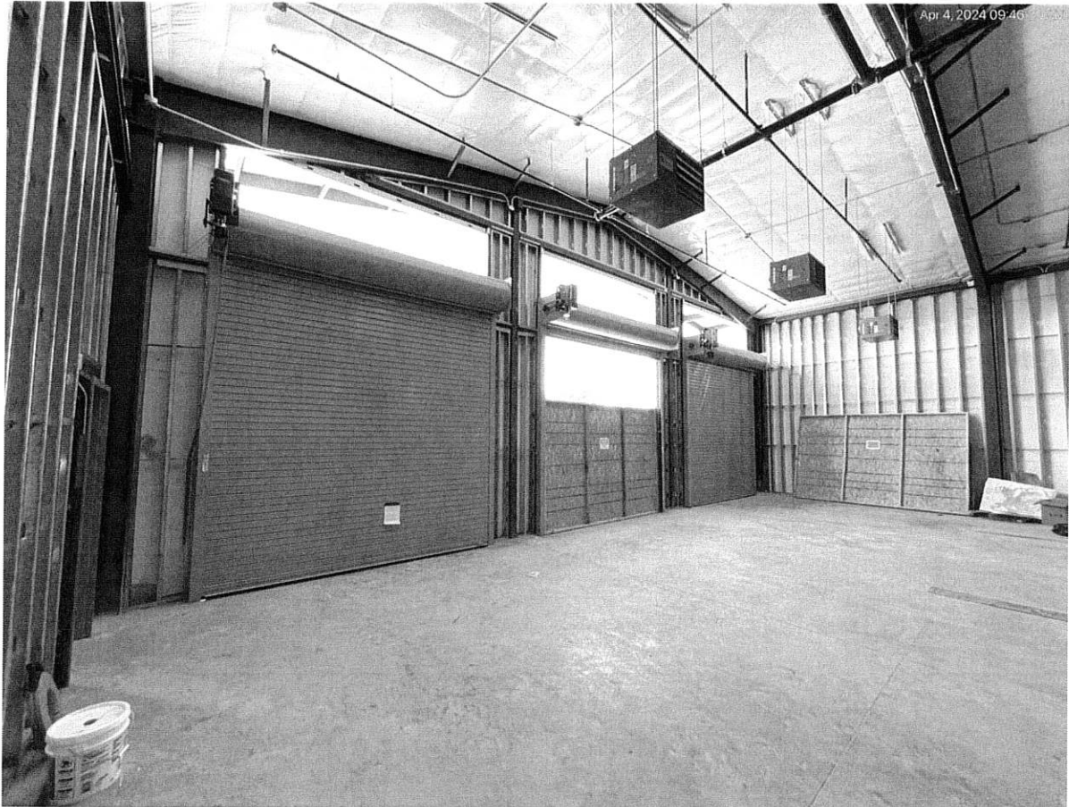
4/4/24 Apparatus bay overhead doors installed
