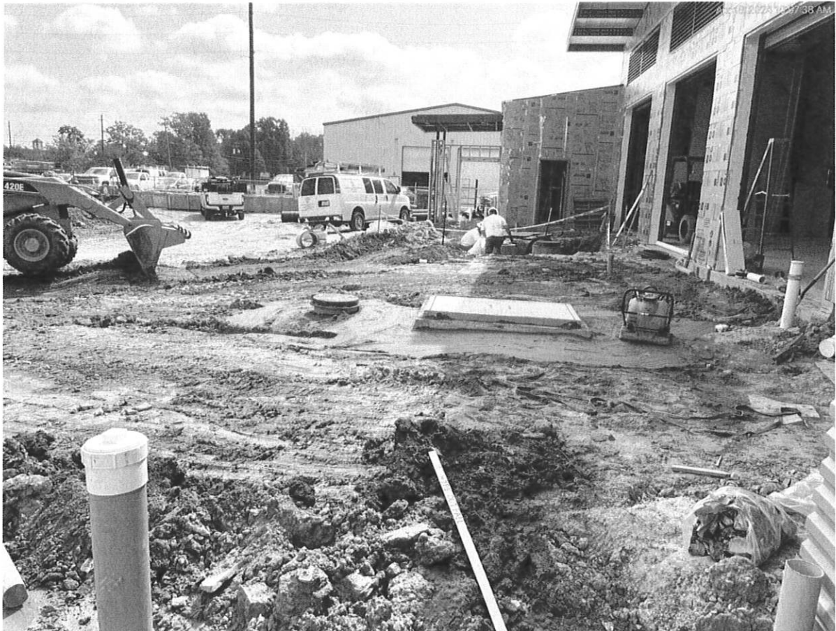
4/18/24 Grease trap and sand/oil separator being installed
