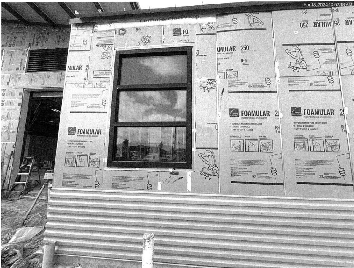
4/18/24 Mockup wall progress overview
