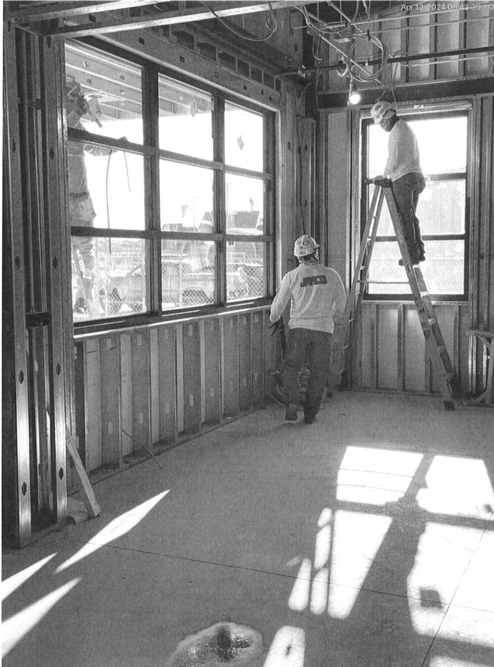
4/12/24 Window install underway
