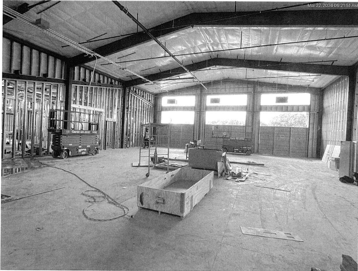
3/22/24 Apparatus bay rough-in progress
