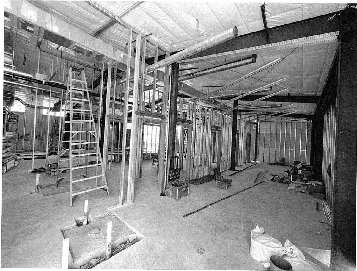
3/7/24 Interior framing and MEP rough-in under way
