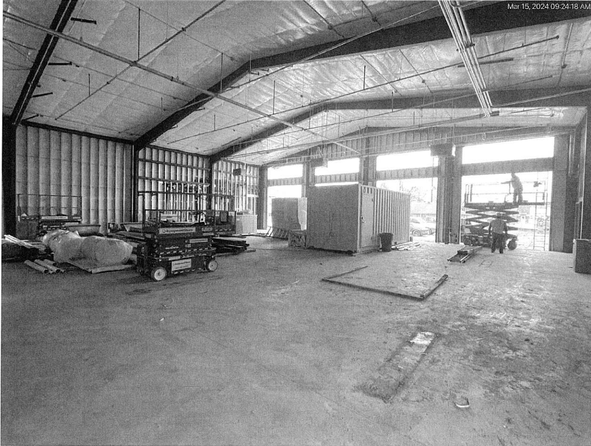
3/15/24 Apparatus bay progress
