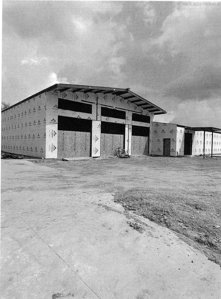
3/4/24 Exterior sheathing completed
