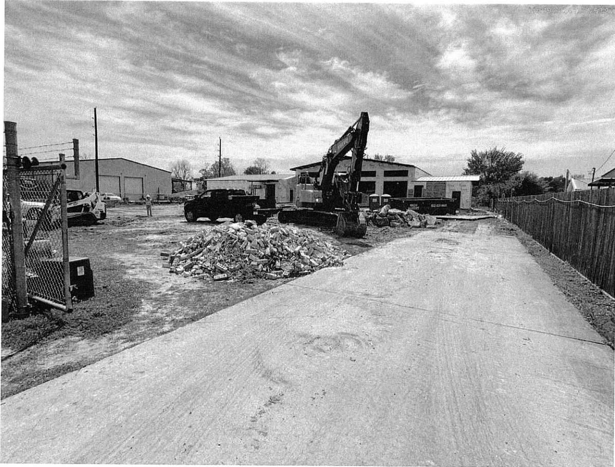
3/19/24 Existing structure demo completed
