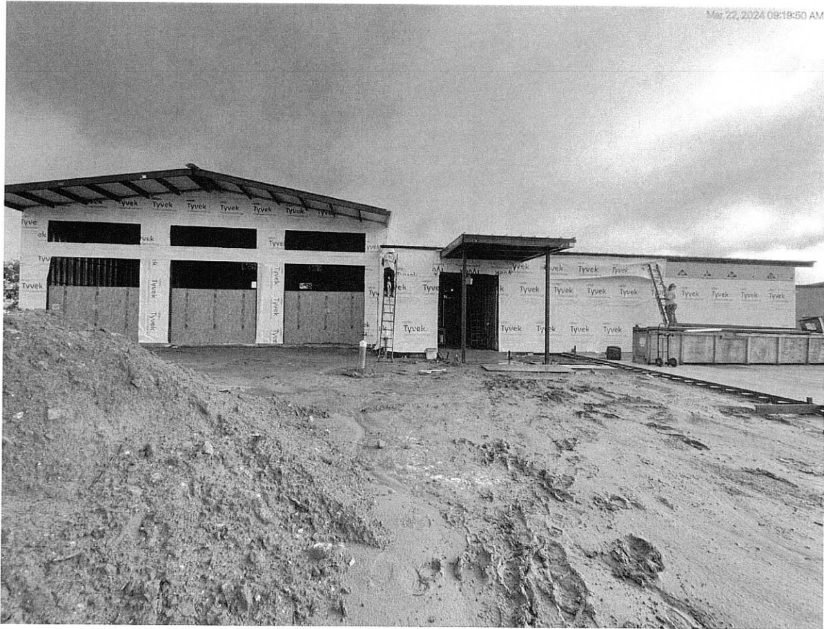
3/22/24 Exterior damp proofing underway
