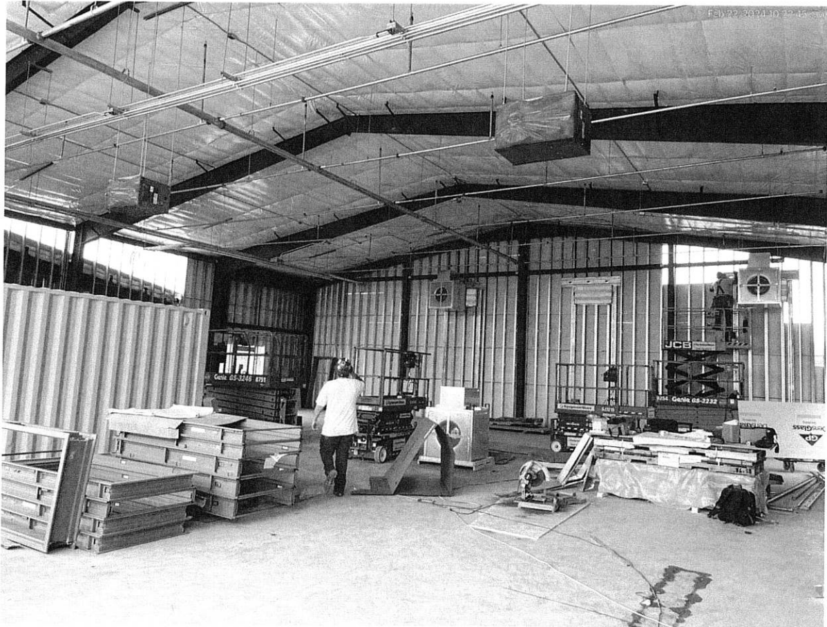
2/22/24 Apparatus bay progress
