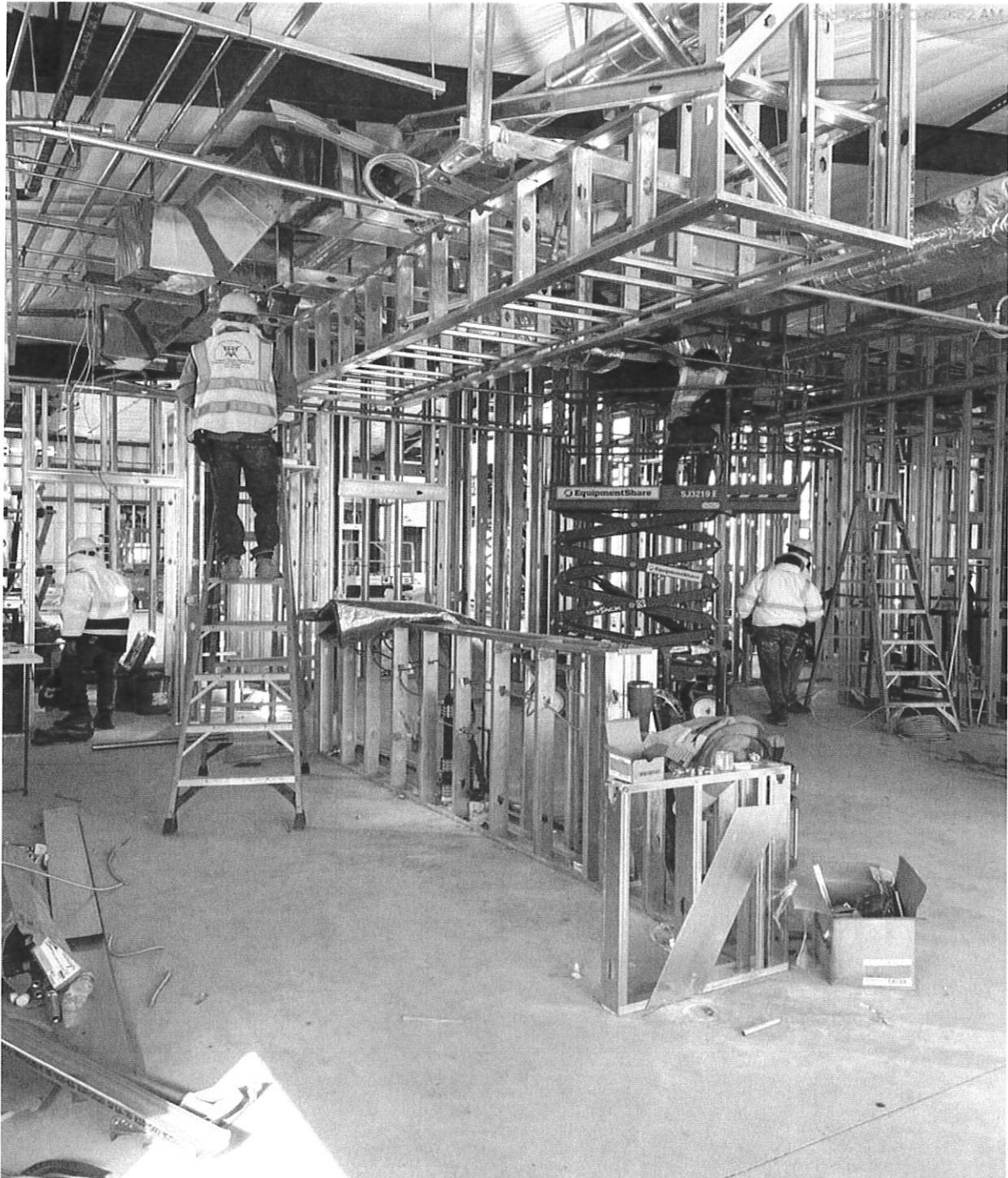
2/9/24 Kitchen area MEP rough-in underway
