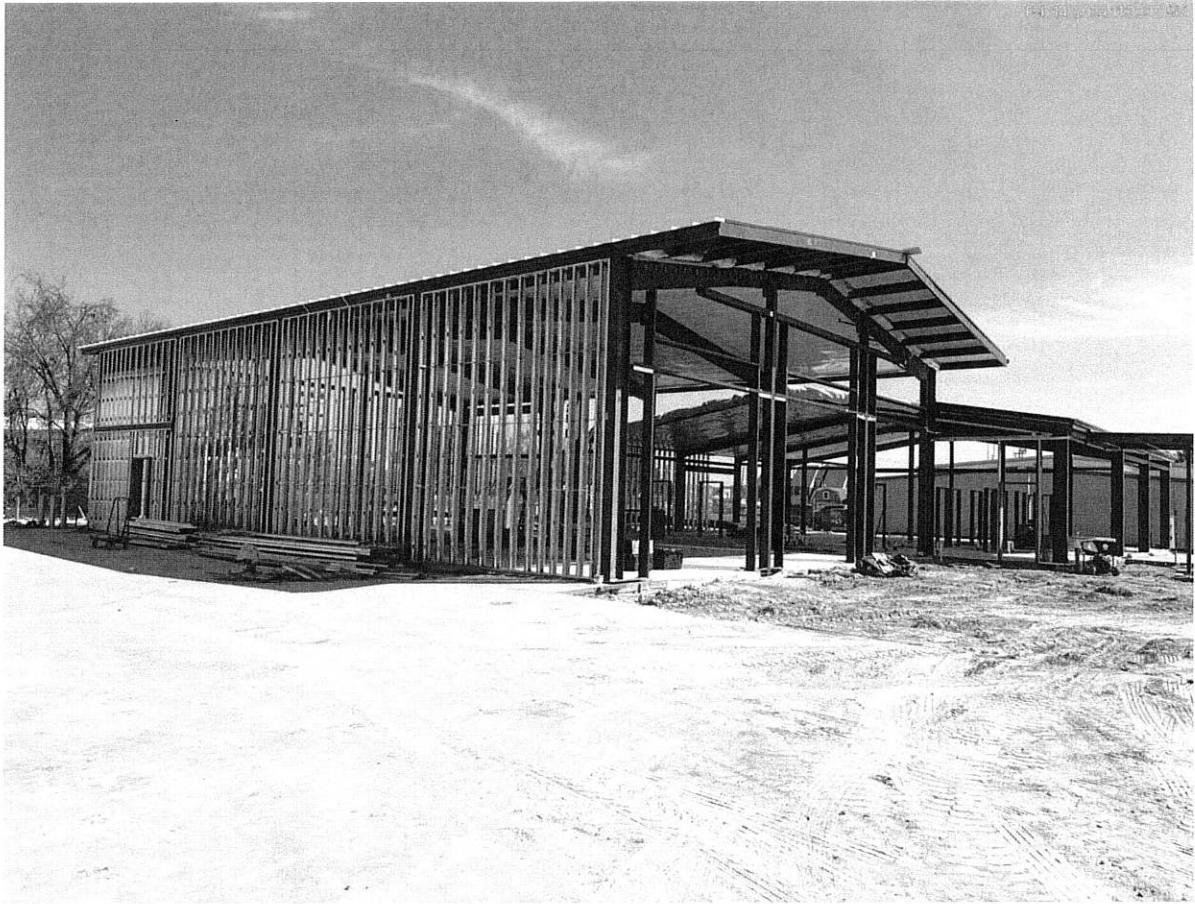
2/14/24 Exterior framing underway
