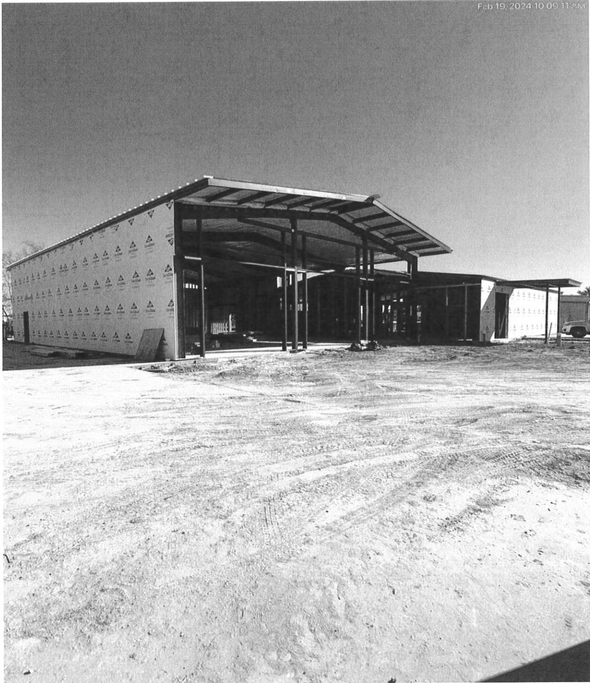
2/19/24 Exterior sheathing underway
