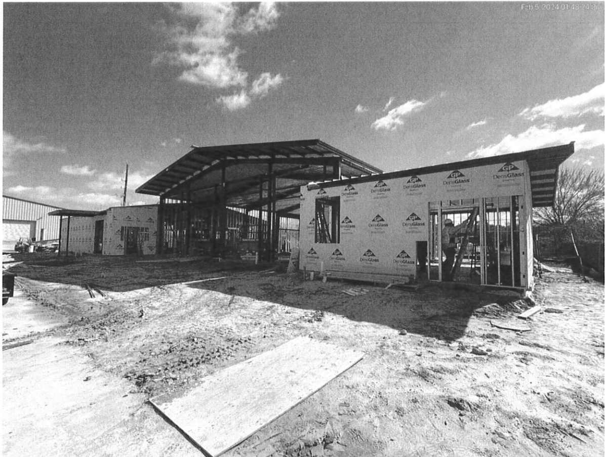
2/5/24 Exterior framing/sheathing underway
