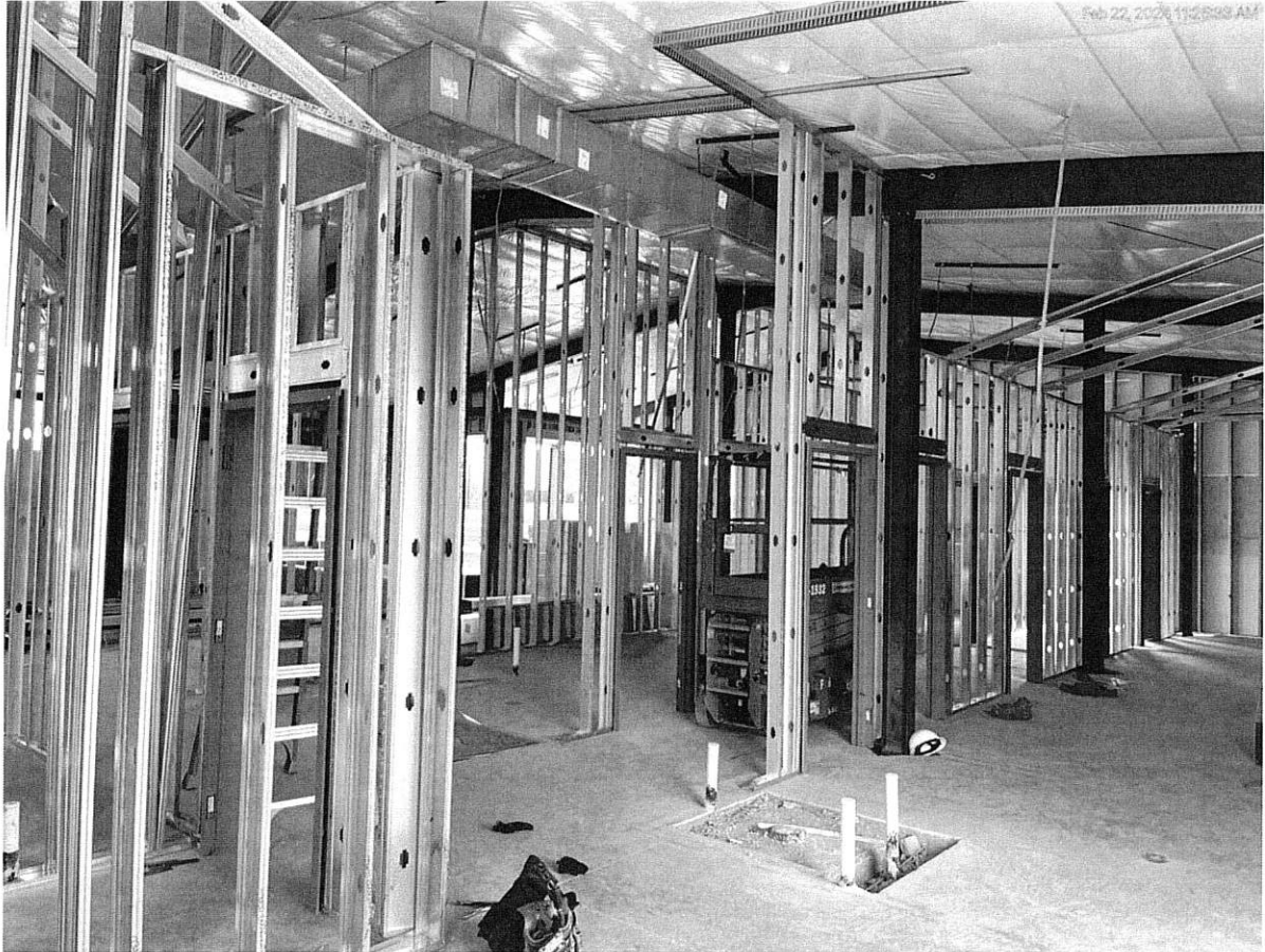
2/22/24 Interior framing progress in the dorm area
