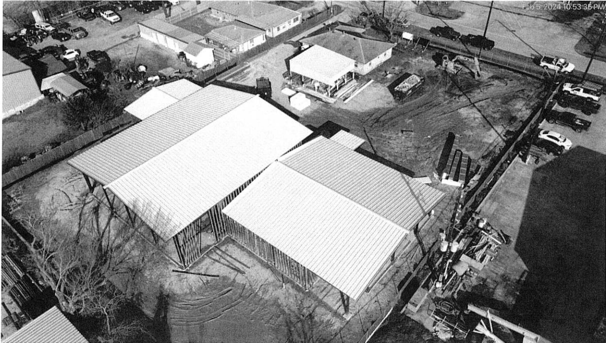
2/2/24 Drone photo overview of site
