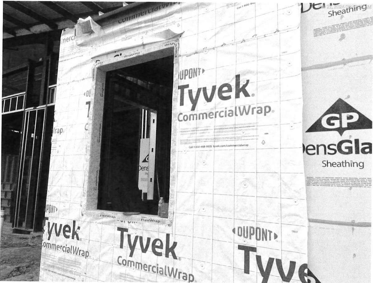
2/22/24 In-place mockup progress
