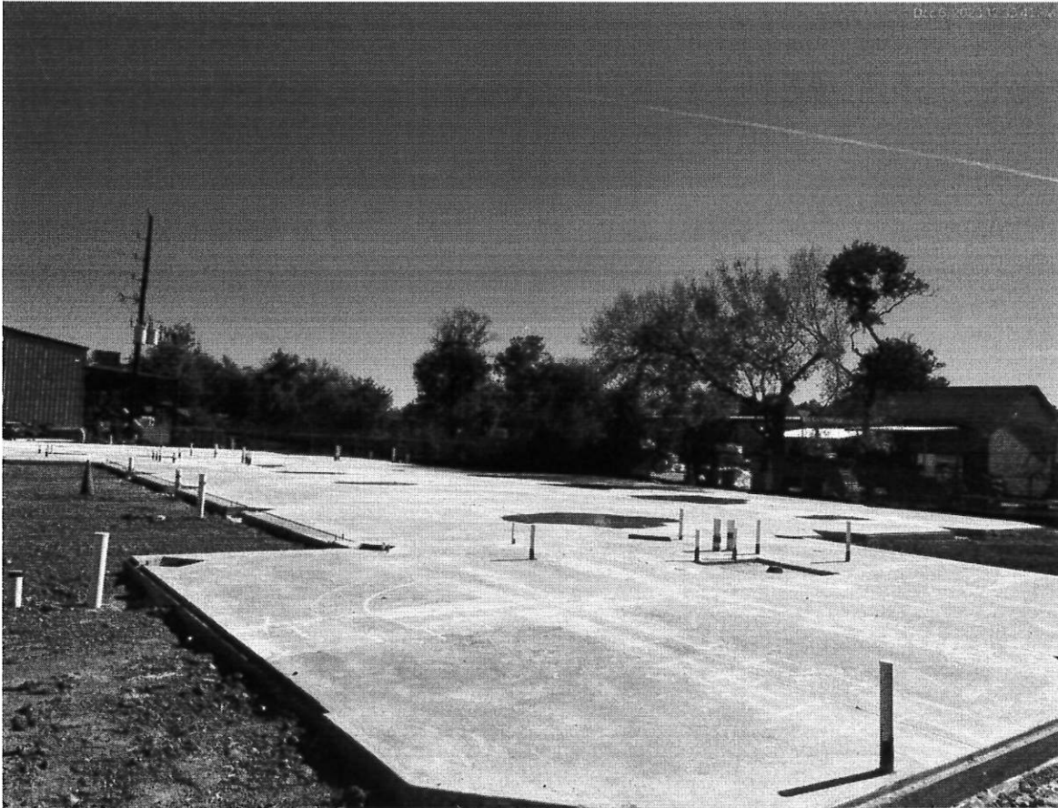
12/6/23 View of the building foundation
