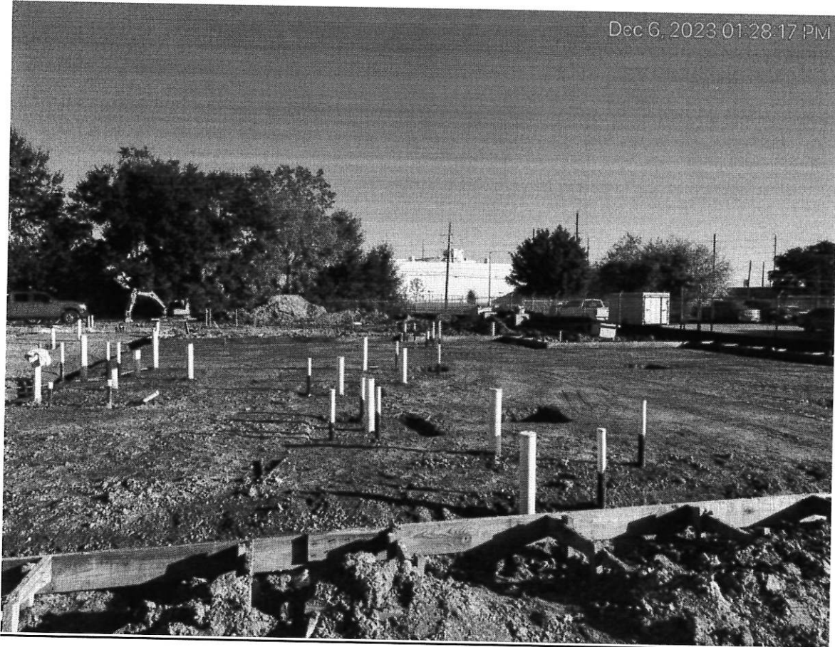
12/6/23 Underslab termite treatment applied
