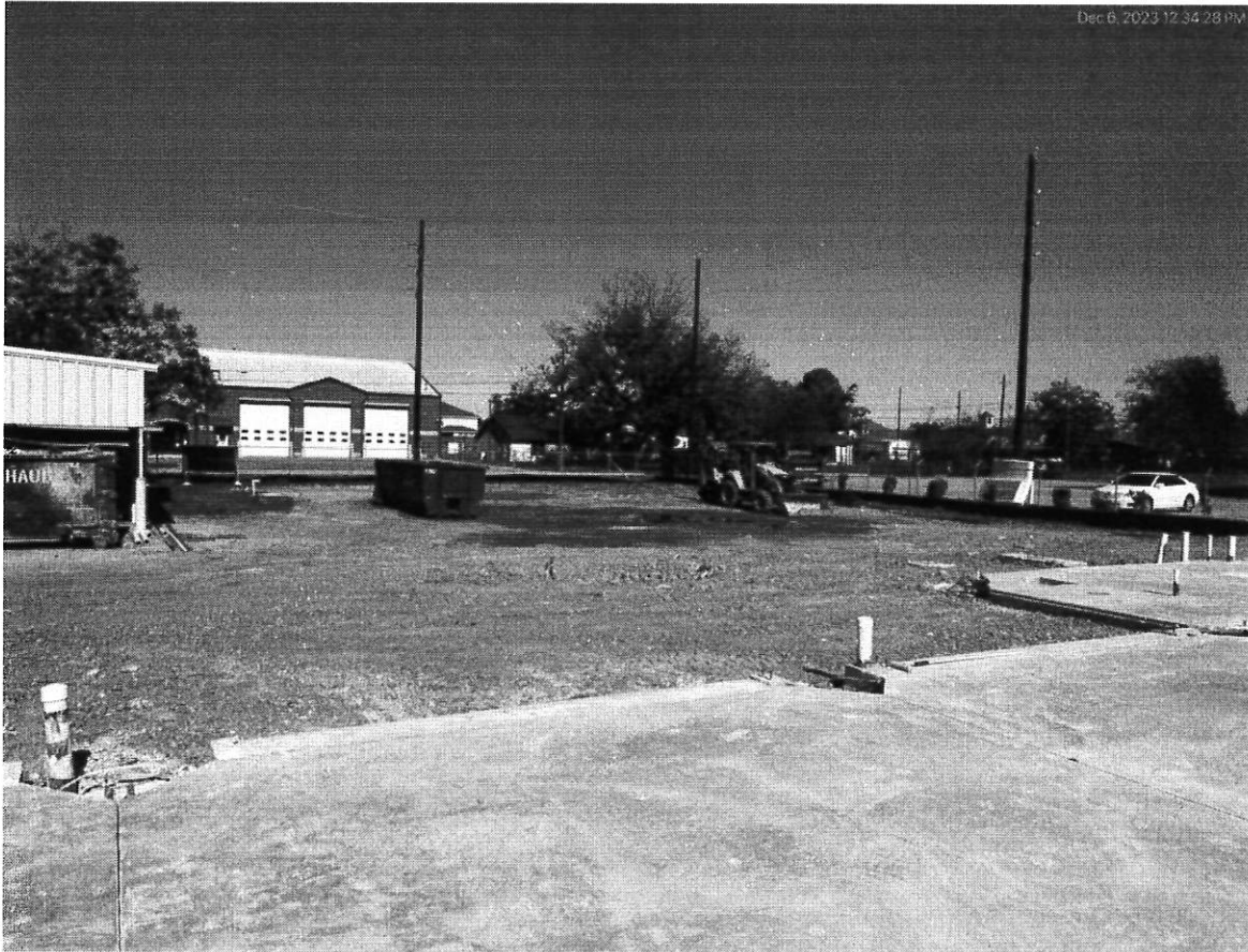
12/6/23 View of the site/detention pond area
