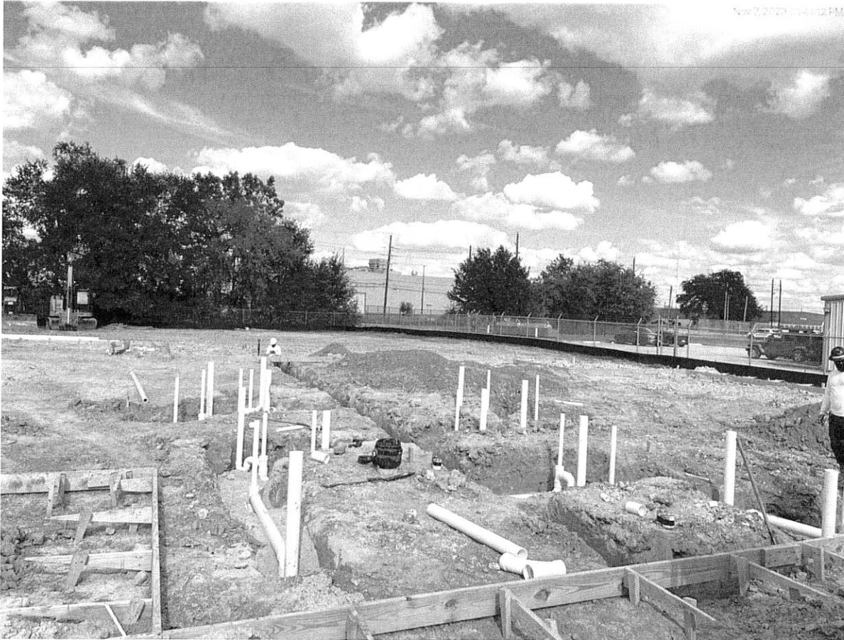
11/7/23 Underslab plumbing installation underway
