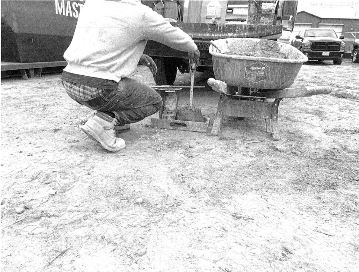
11/9/23 Foundation grade beam slump test
