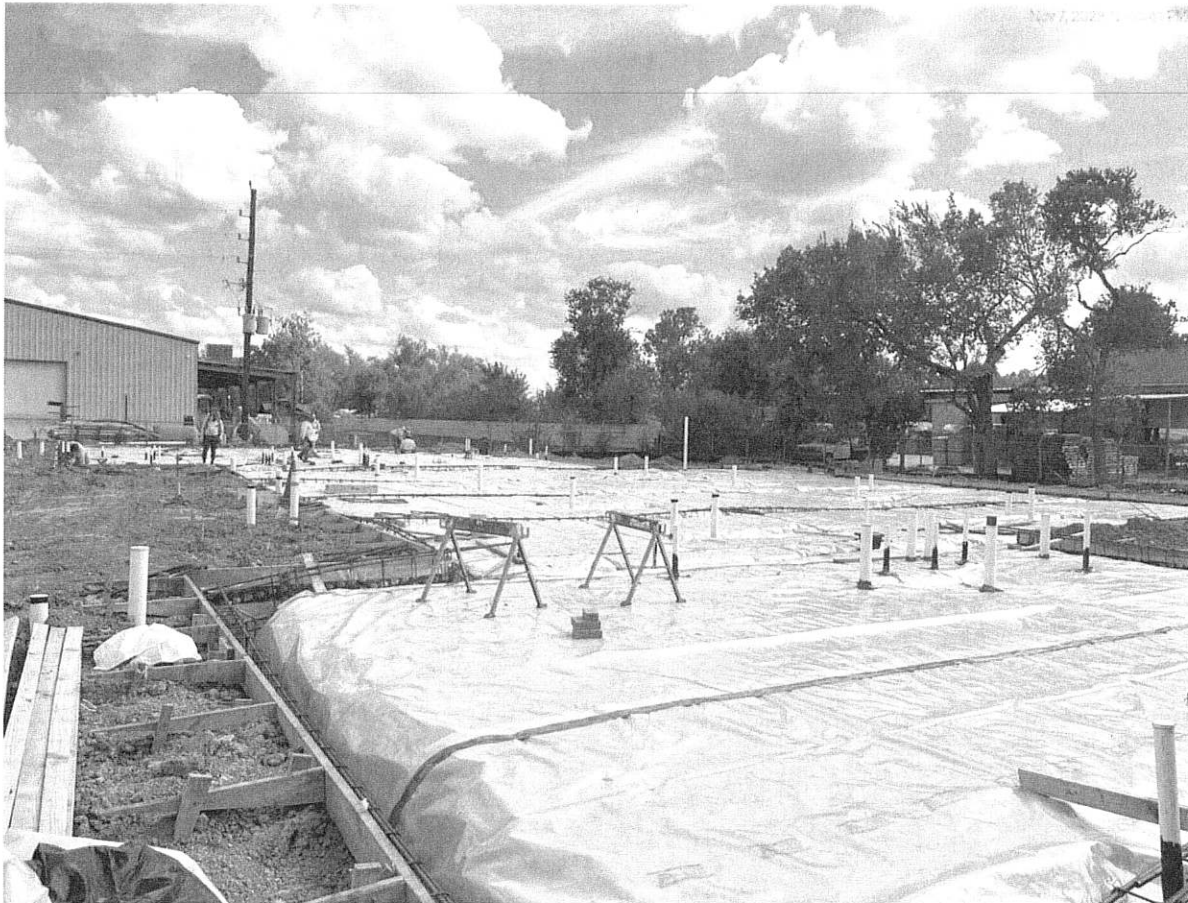
11/7/23 Foundation vapor barrier and rebar installation underway
