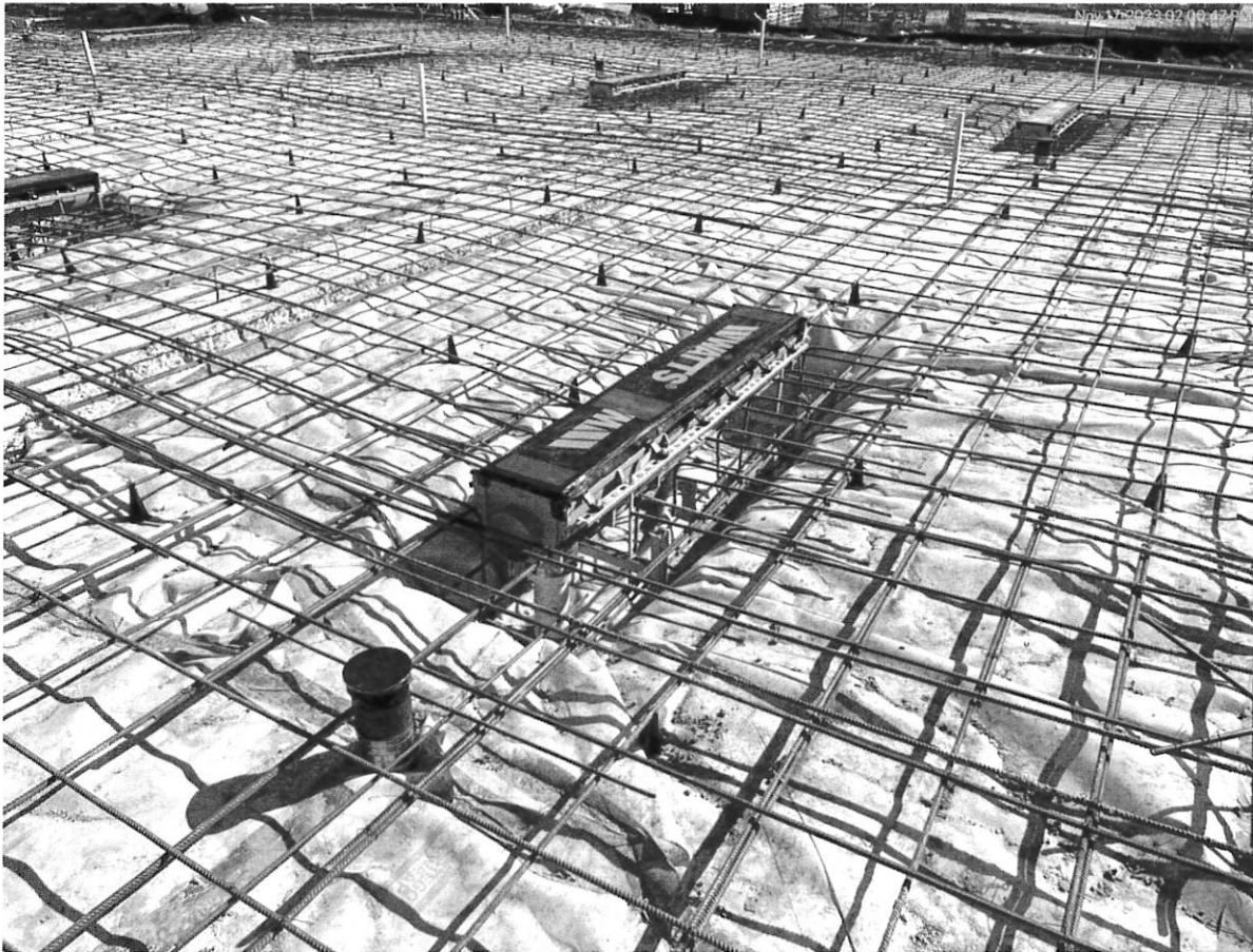
11/17/23 Trench drain installation (typical)
