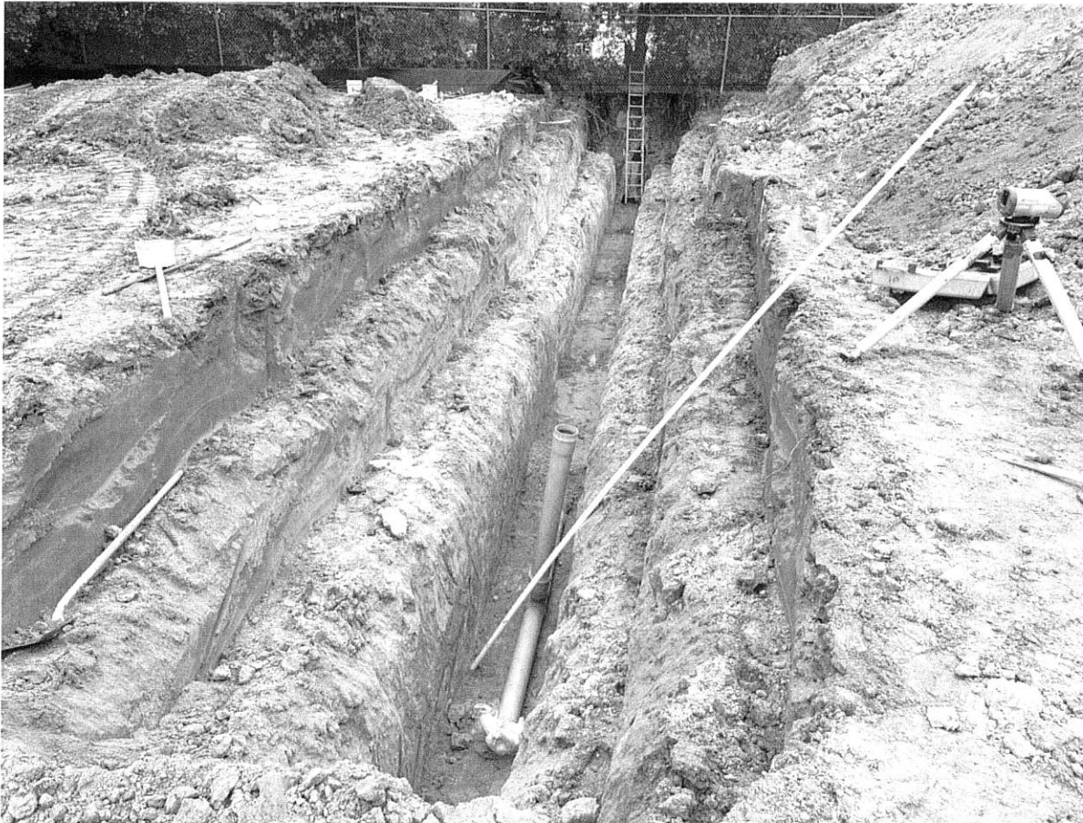
11/17/23 NW site excavation and sewer installation
