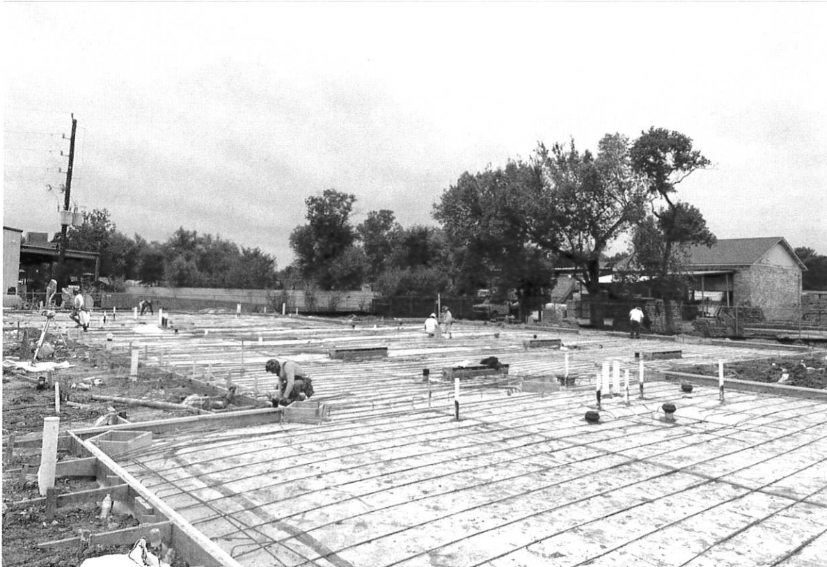
11/16/23 Foundation rebar installation
