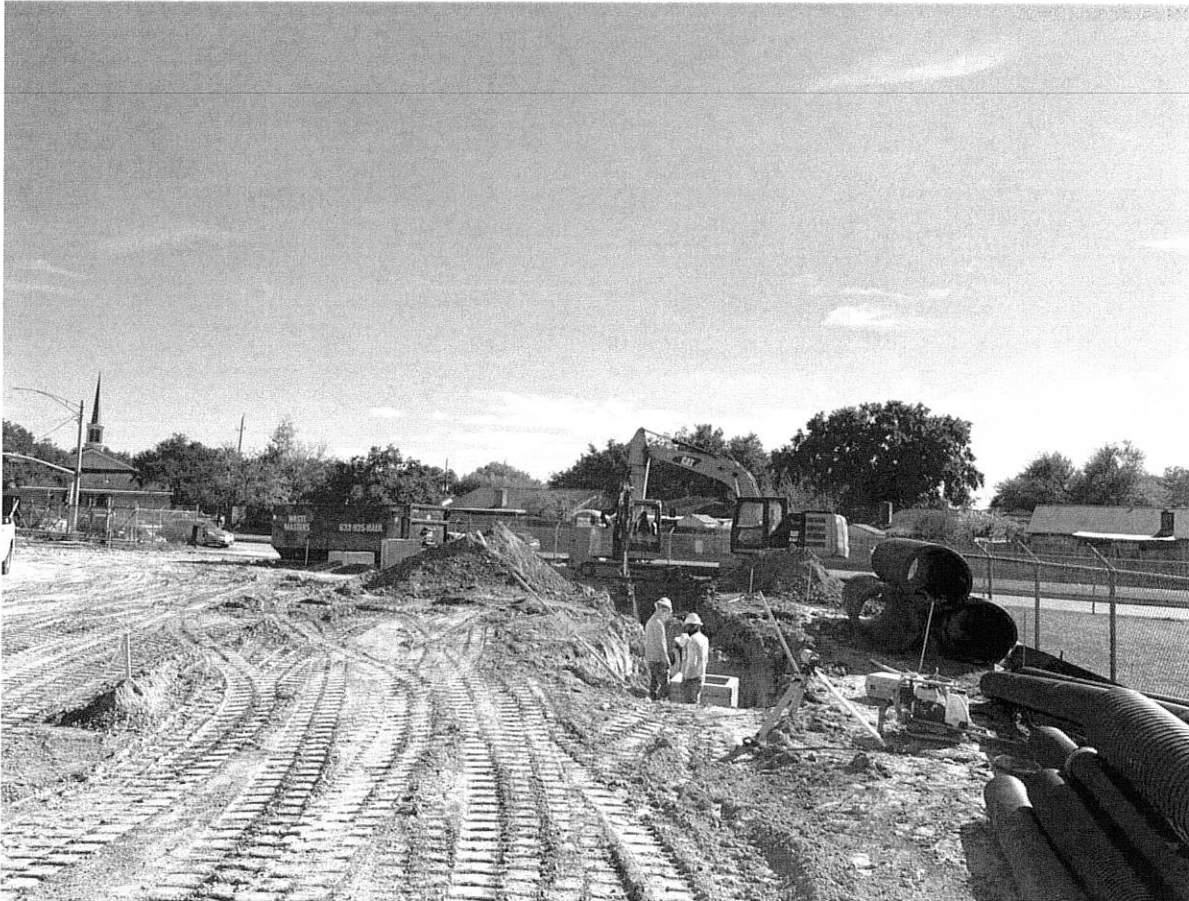
11/17/23 SW storm sewer excavation and installation
