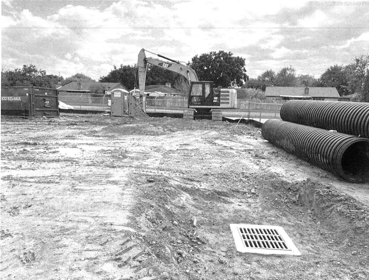
11/20/23 SW site storm drain installation complete
