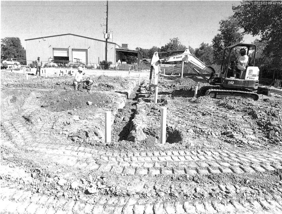
11/1/23 Underslab plumbing excavation and installation
