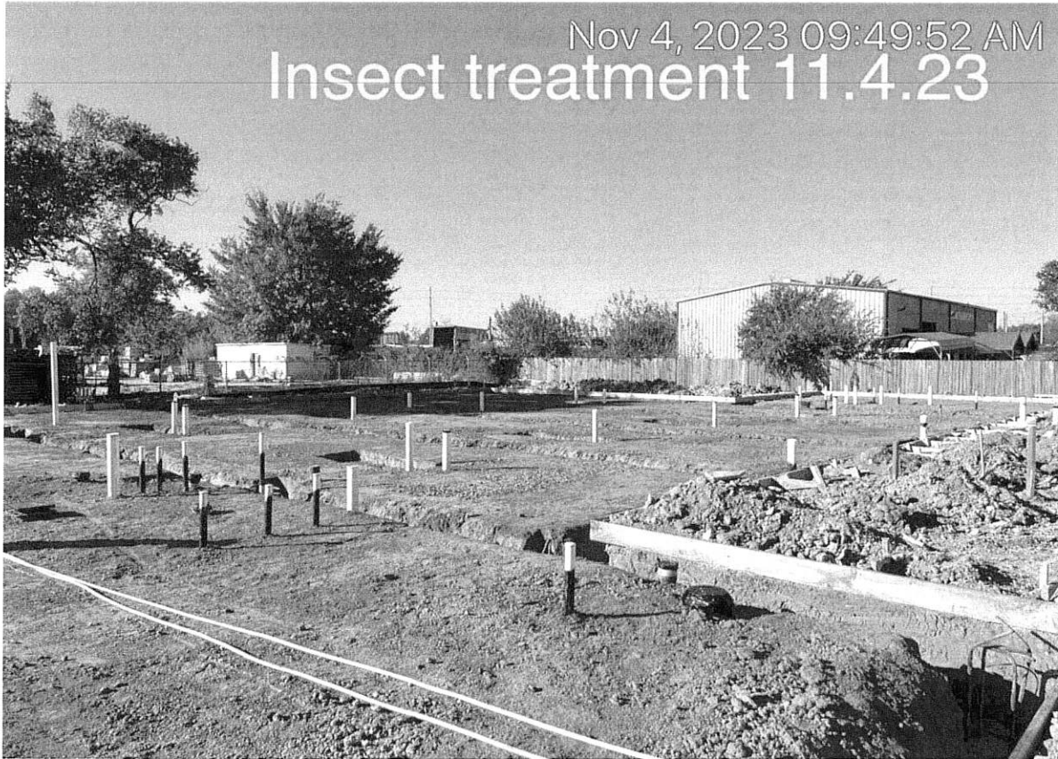
11/4/23 Foundation termite treatment
