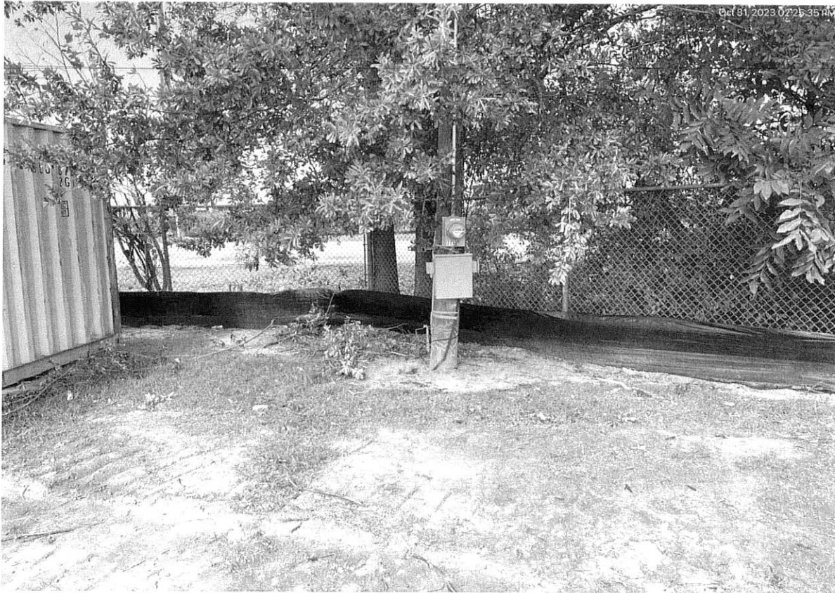
10/31 Temporary power meter installed
