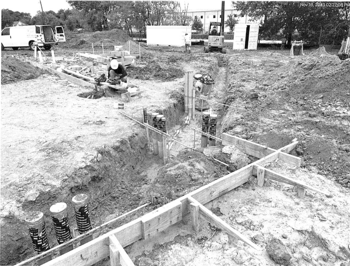
11/16/23 Underslab and site electrical installation underway
