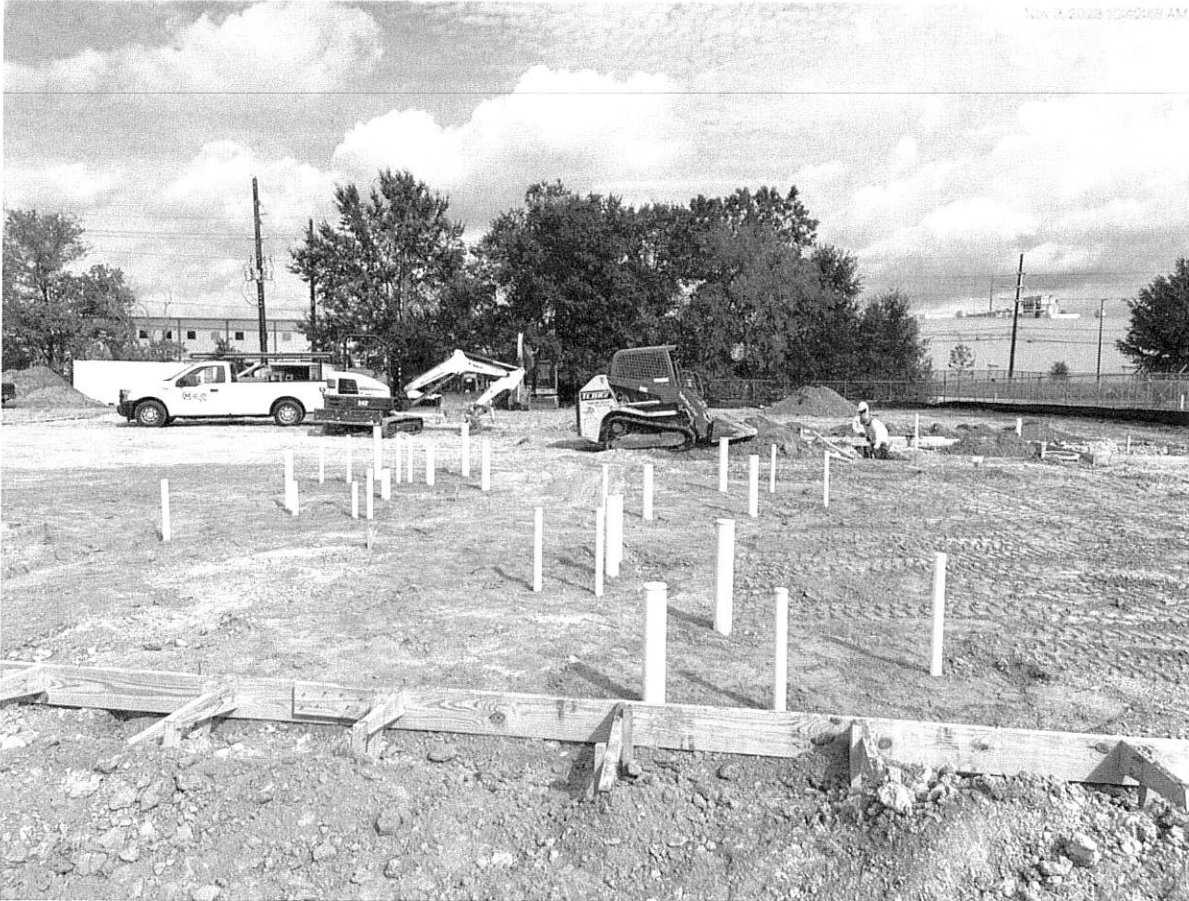
11/9/23 Underslab plumbing backfill and compaction
