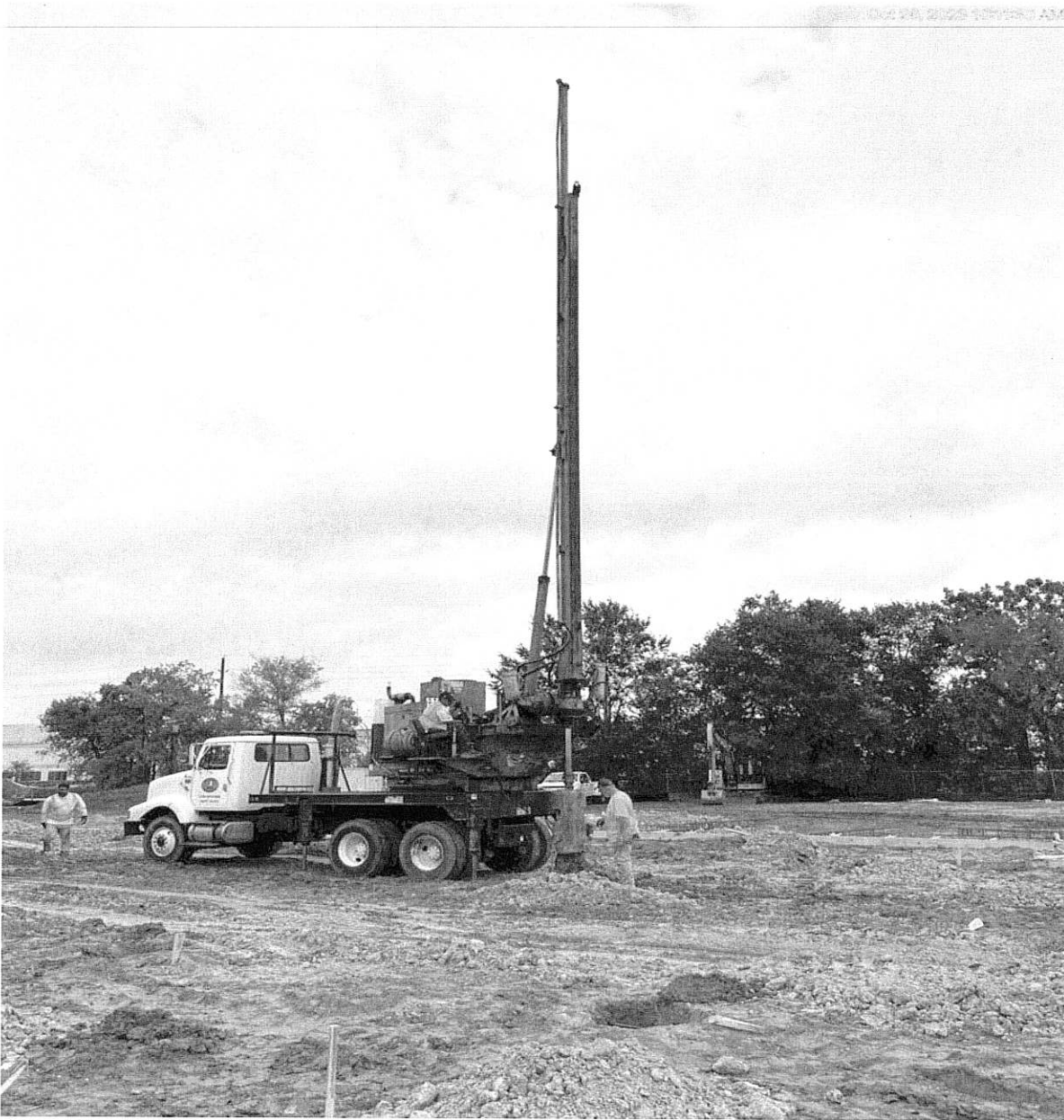
10/26/23 Drilling rig being used to drill all piers
