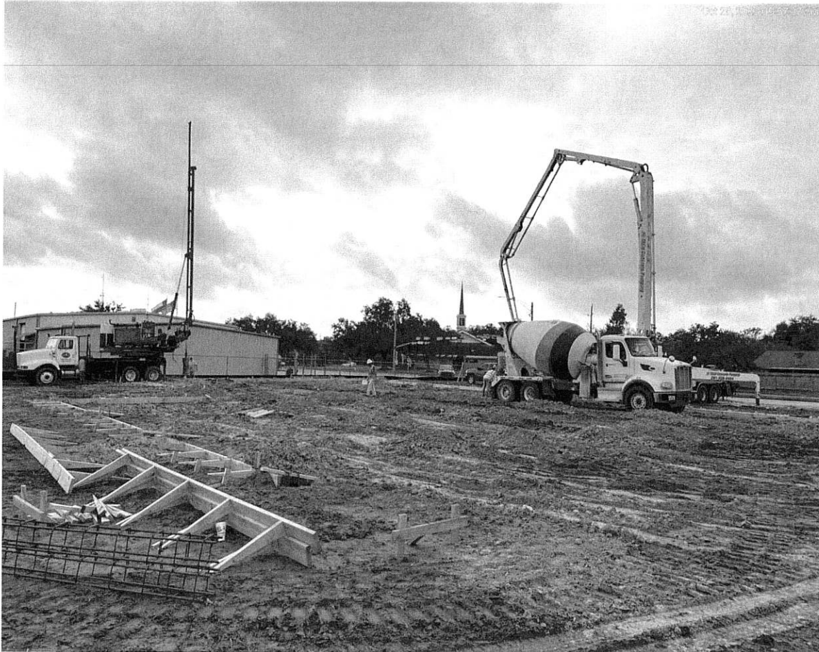
10/26/23 Pier drilling and concrete pour underway
