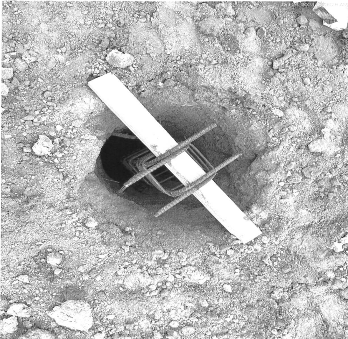
10/26/23 Drilled pier and rebar (typical)
