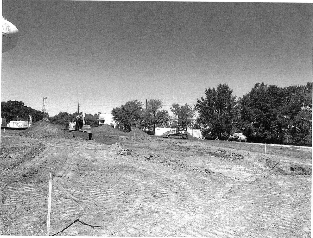
10/20/23 Building pad prep underway
