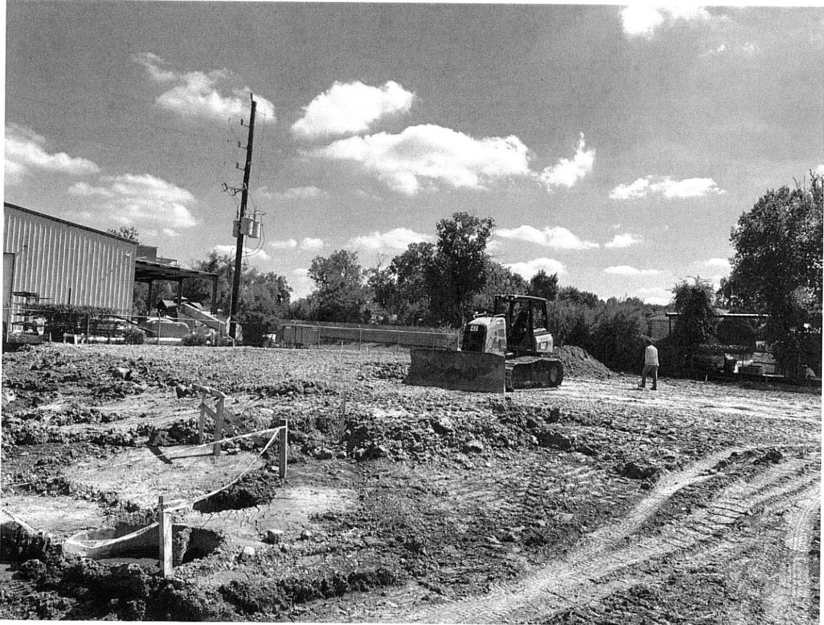
10/12/23 Building pad importing/spreading/leveling underway
