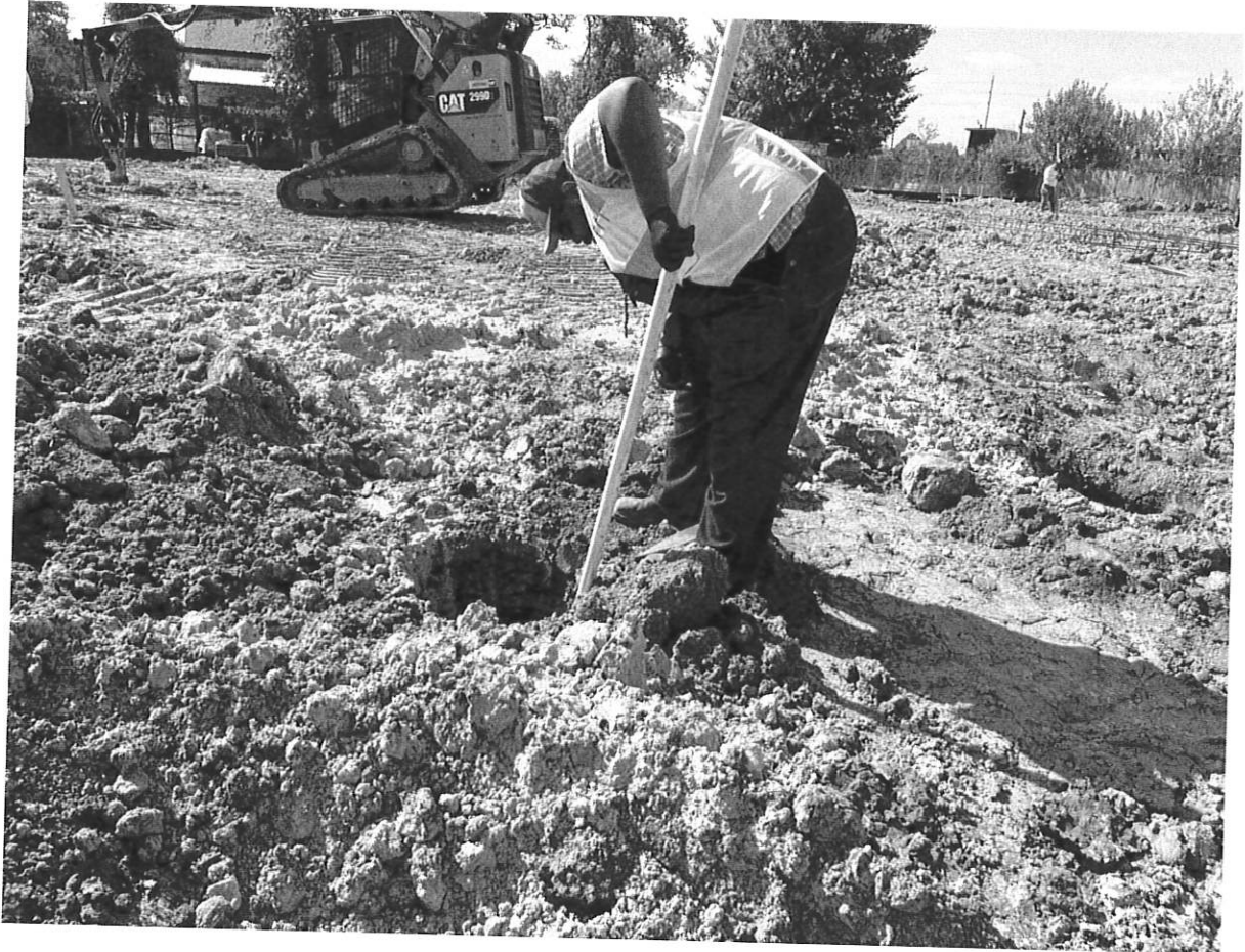
10/13/23 Pier inspection underway
