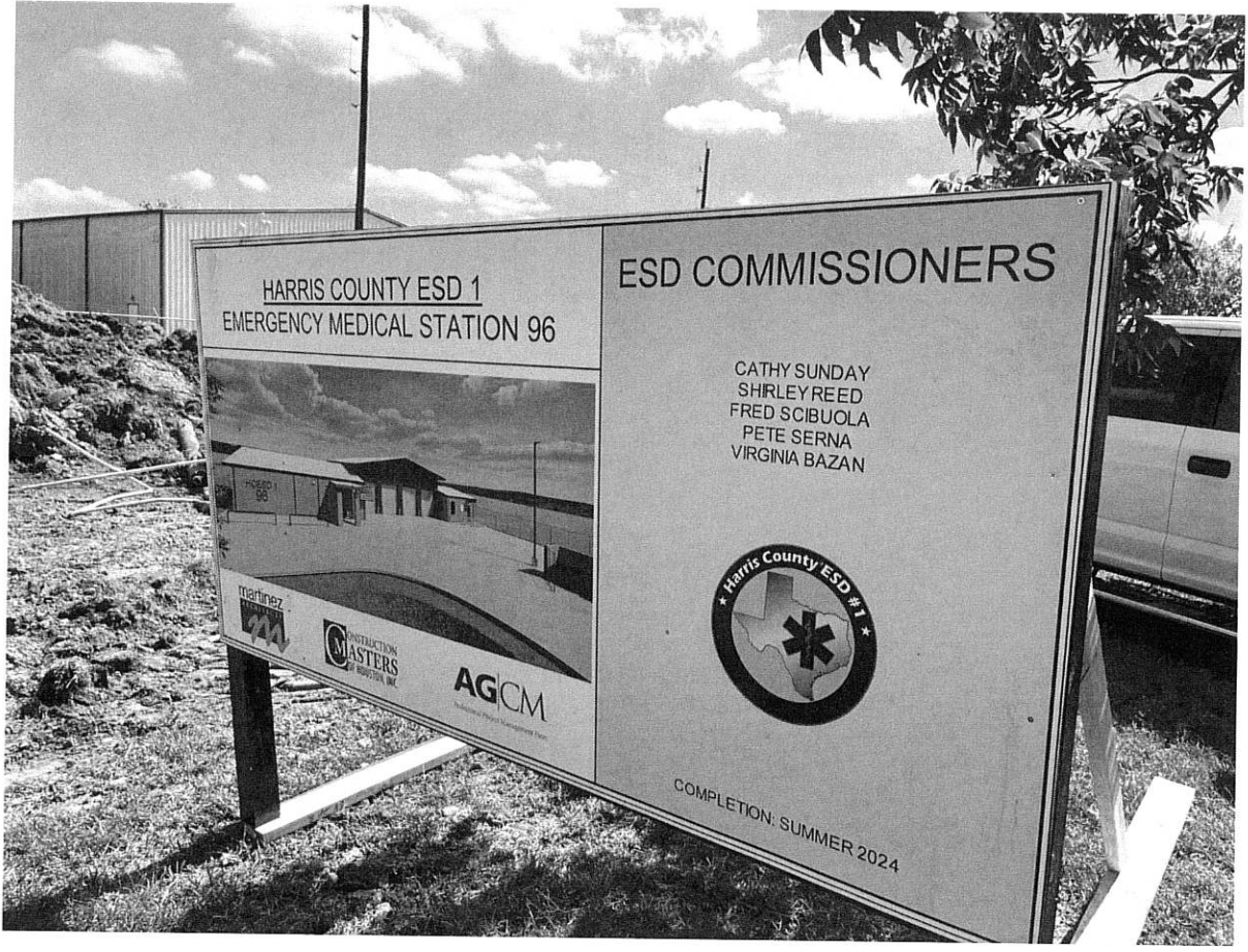
10/12/23 Project sign installed
