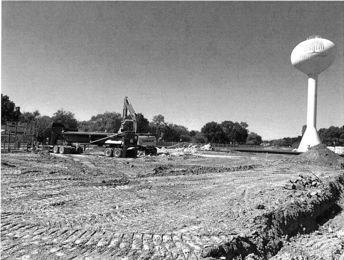
10/20/23 Existing pavement and foundation demolition underway
