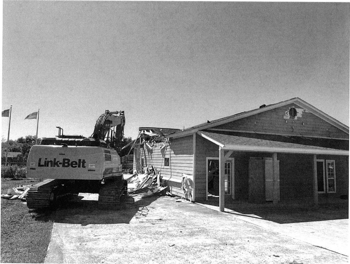
10/16/23 Existing building demolition underway
