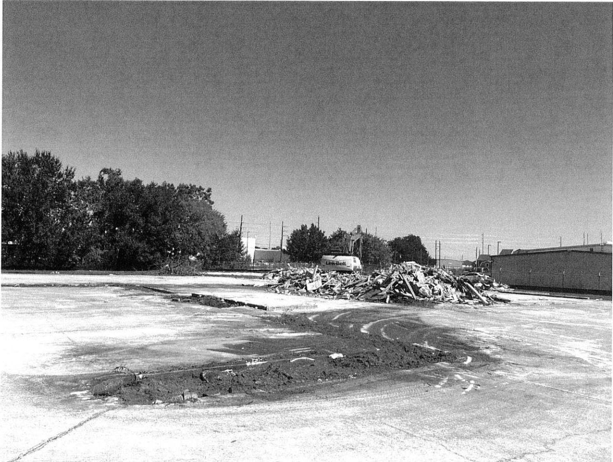
10/17/23 Existing building demolition complete
