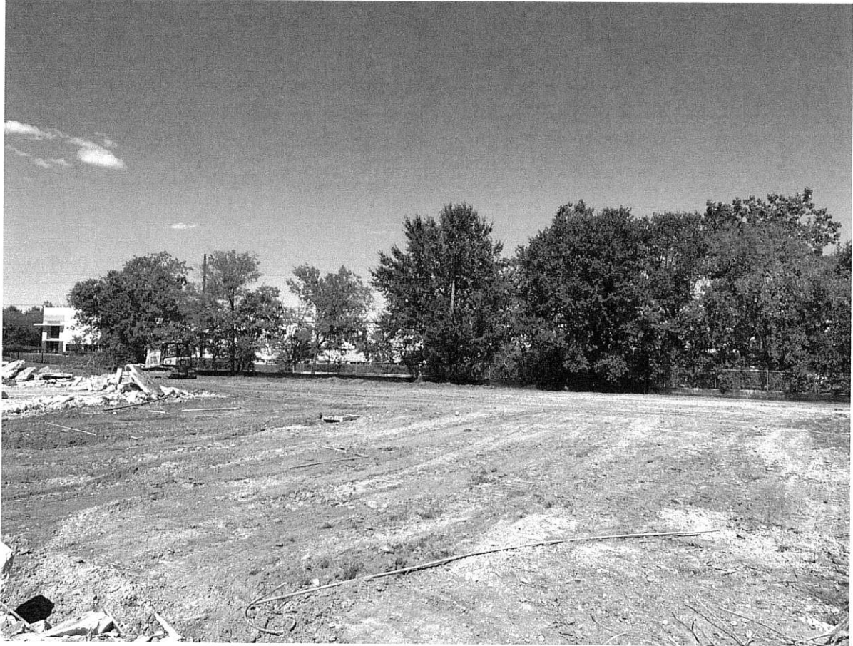
10/18/23 Building pad site scraped
