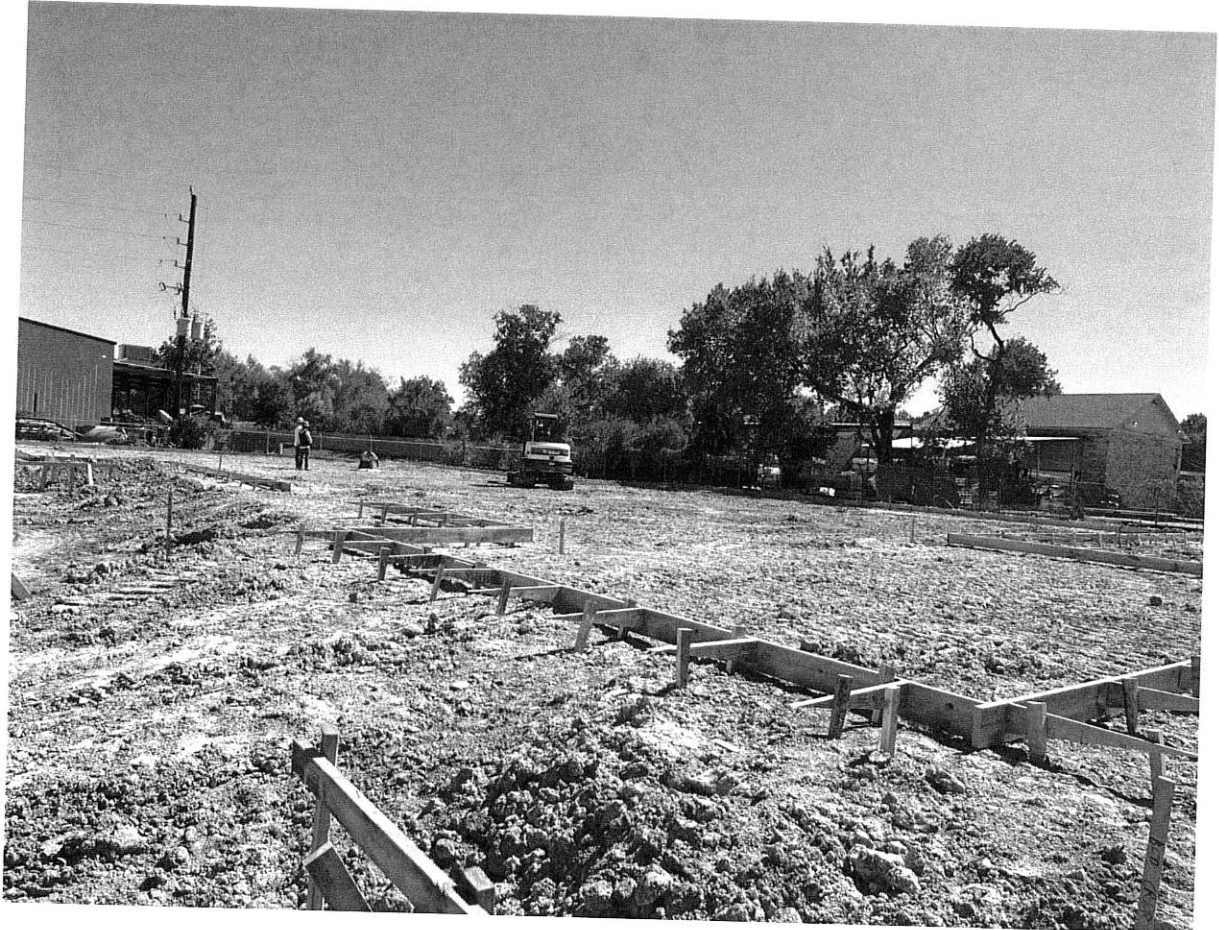
10/16/23 Foundation forms installed
