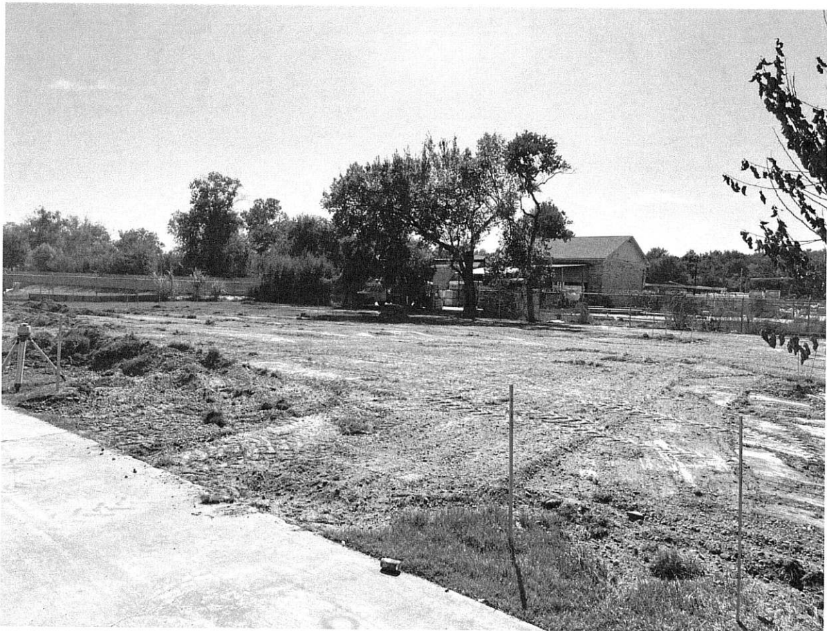
10/2/23 Building pad area scraped
